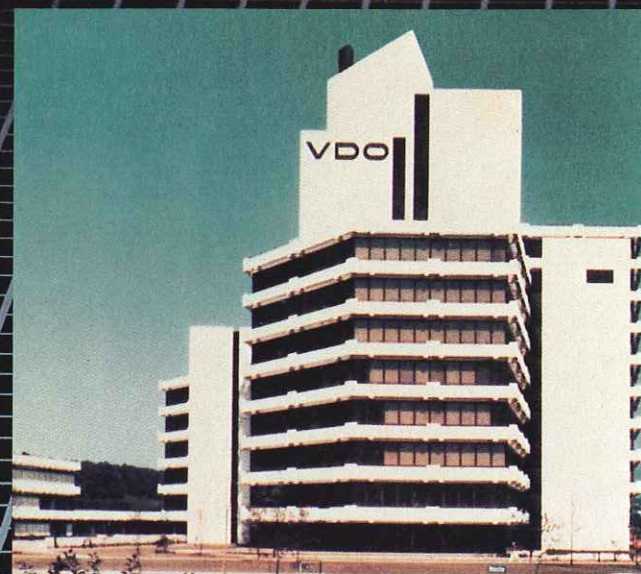
VDO Headquarters and Research & Development Center at Schwalbach, Germany.
