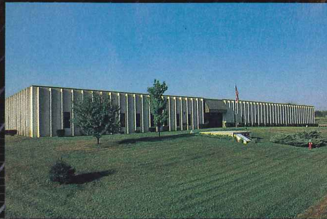
VDO Headquarters including production facilities in Winchester, Virginia.
